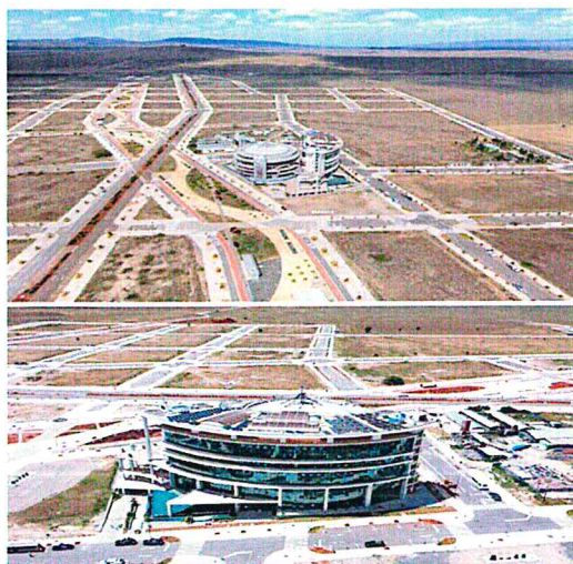
Completed infrastructure and facilities within Konza Technopolis
