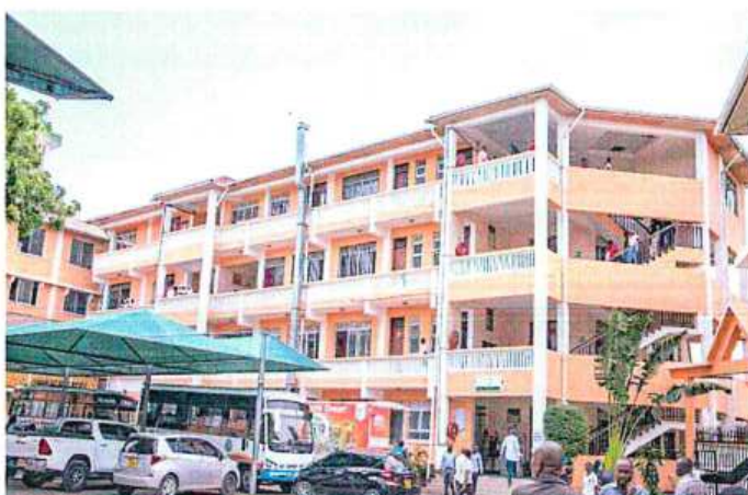
The commissioning of a newly build multi-storey academic block at the Kenya Coast National Polytechnic in Mombasa, 24 February 2026
