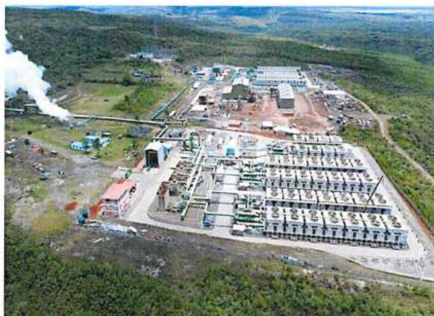
35MW Orpower 22 Geothermal Power Plant at Menengai, Nakuru County.
