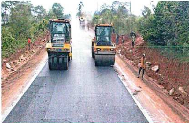
Ongoing upgrading of the Ainapsetan–Chepterwai Road in Nandi County
