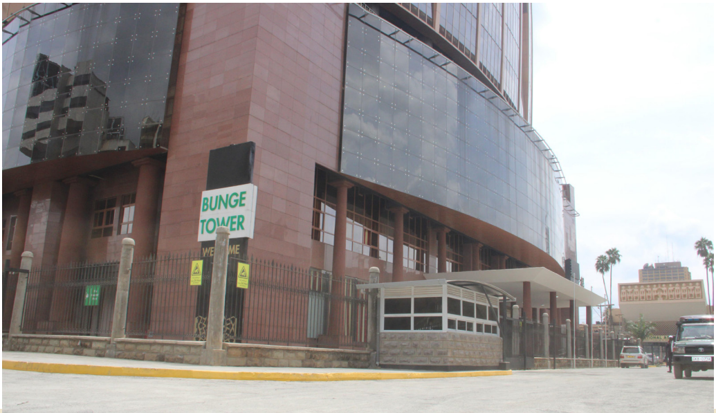
Recarpeting outside Bunge Tower entrance
