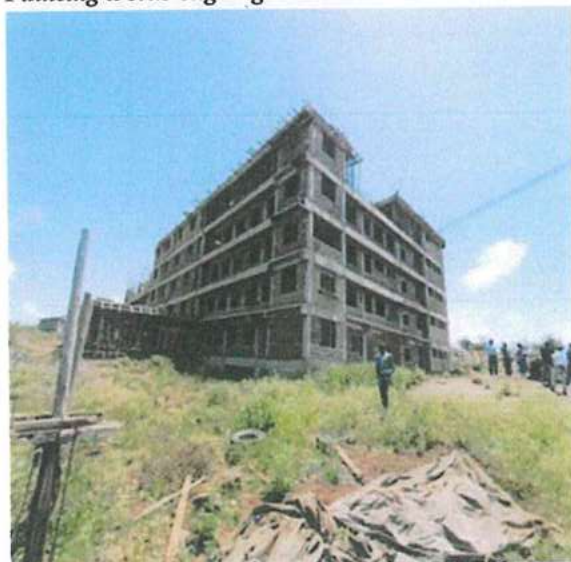
Ongoing Construction of Marsabit High court
