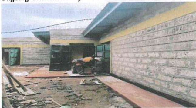
Painting works ongoing in Karatina cell block
