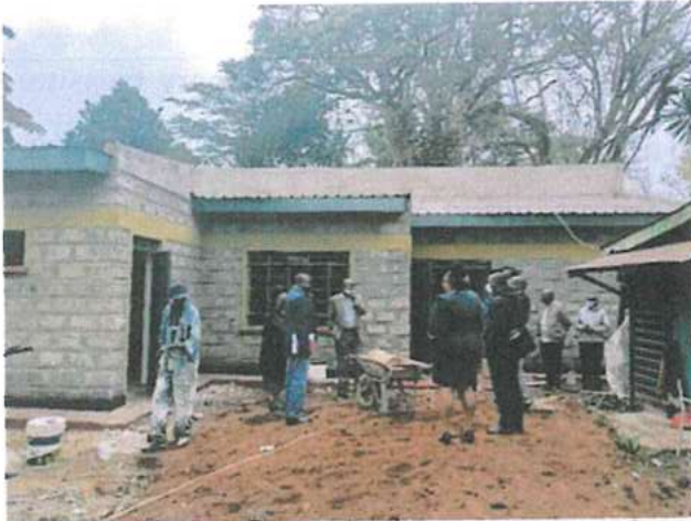
Ongoing Construction of Cell Block in Karatina
