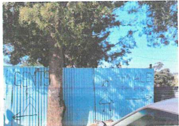
Old Toilet at Iten Law Court
