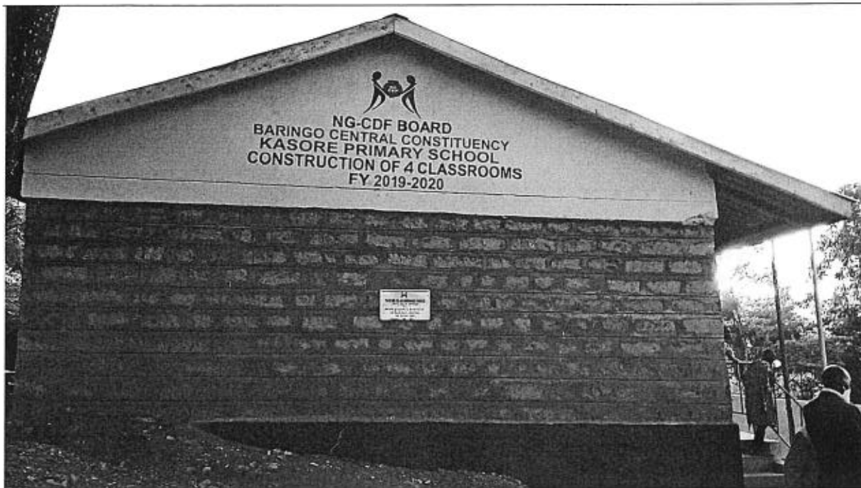
Kasore Primary School Construction Of 4 Classrooms
