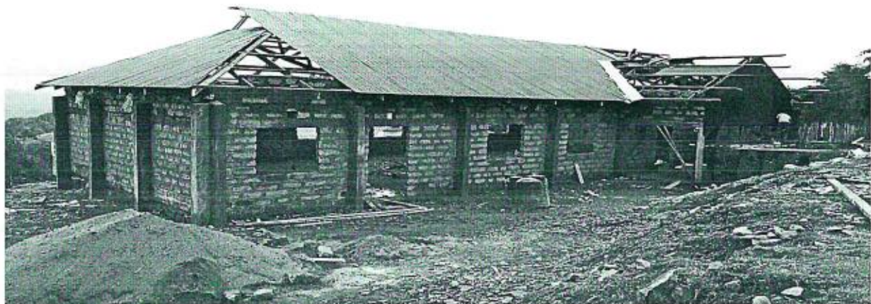
Kapsogo Day Secondary School- Ongoing Construction Of Multipurpose Hall
