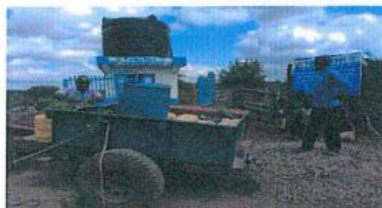
Sokomoko Borehole funded by GoK through National Water Harvesting Programme
