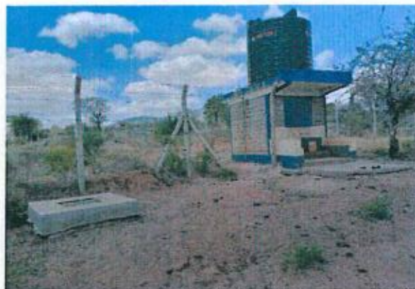
Nuu Special School Water Kiosk Constructed under drought mitigation programme
