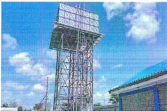
Mavoko Drinking Water Project- Syokimau_300m3 Elevated tank
