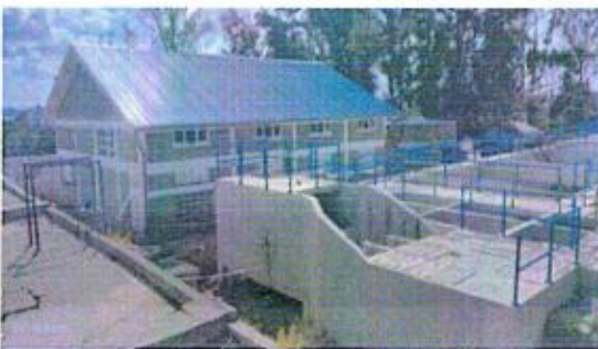
Mavoko Drinking Water Project- WTP_Chemical Building and Mixing Chamber
