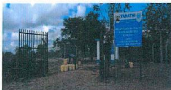
Wananchi taking water from Kavisuni Borehole Water Project constructed under the Drilling & Equipping 40No. Boreholes funded by GoK
