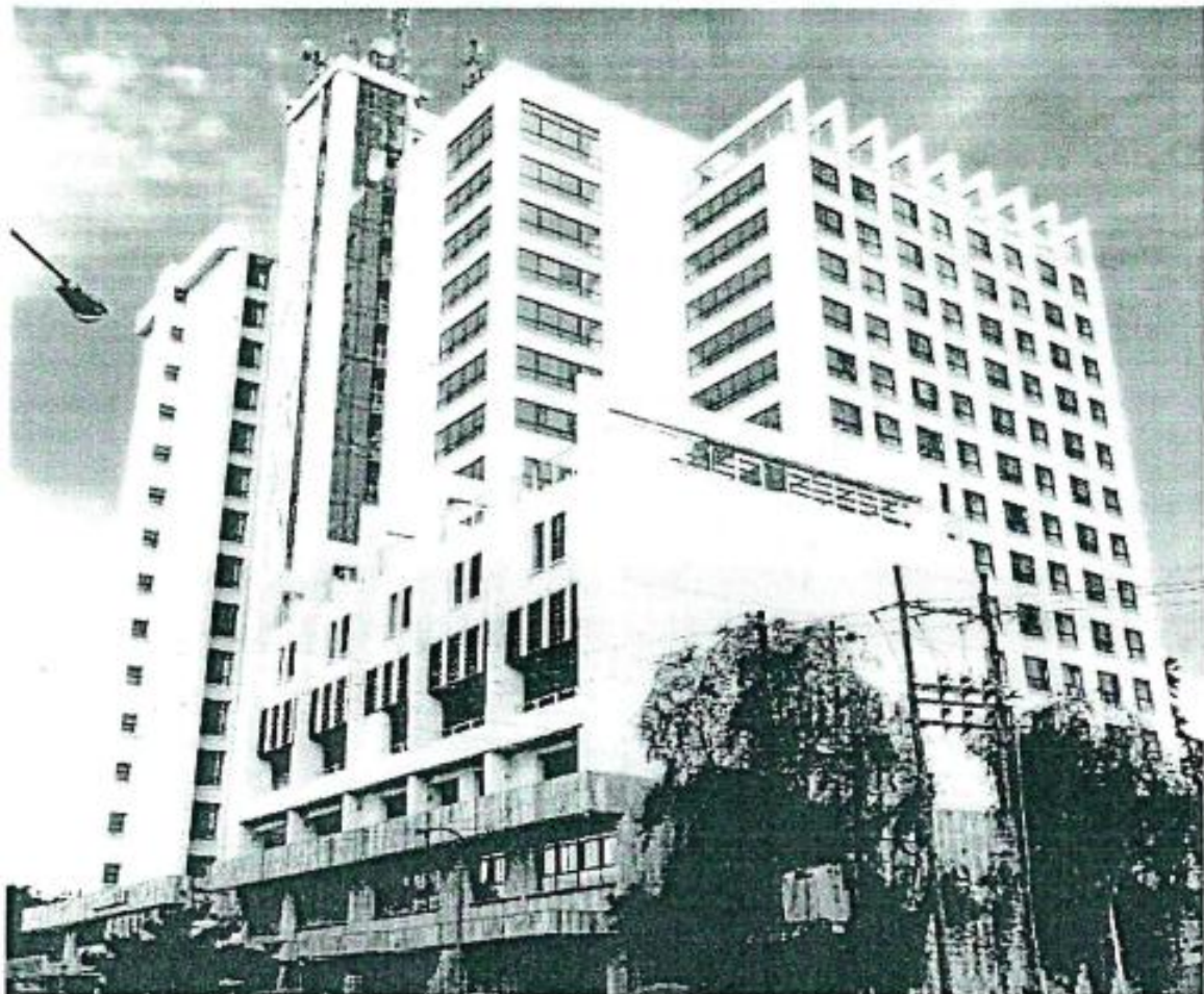
KVDA Complex in Eldoret
