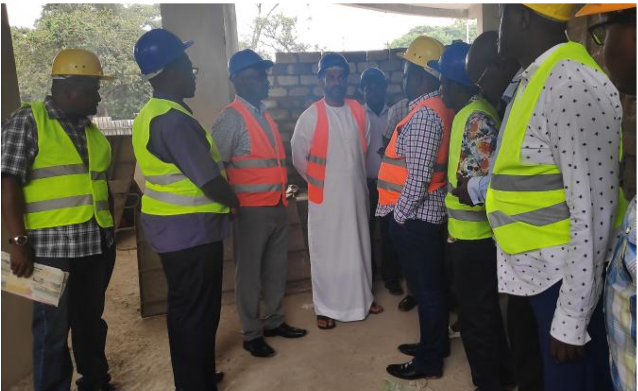
Members of Public Investments Committee inspecting the stalled construction of Kenya Maritime Authority office building
