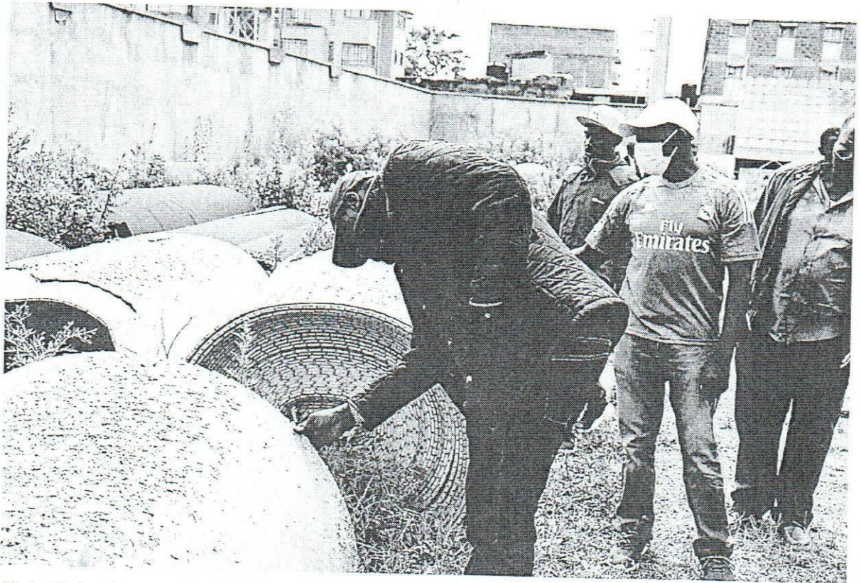
Photo 5 showing part of the artificial grass turf and other equipment going to waste. The stadium has so far costed Ksh 123million of the Ksh 350 million earmarked for Dandora Stadium
