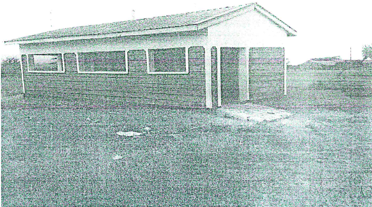
Olesharo Girls Secondary School Toilets- Ongoing painting works.
