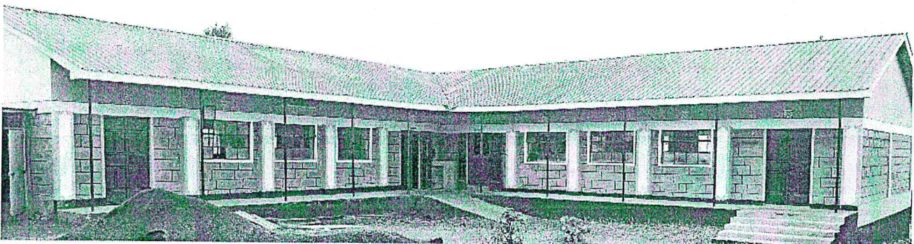
Mwiruti secondary school- Construction of twin laboratory
