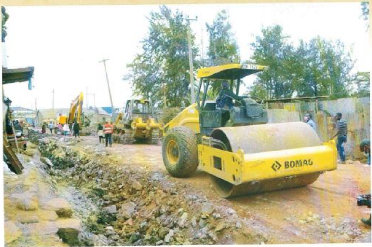
Bulldozer compacts a road in Mukuru Kwa Njenga (Photo by KNA)
