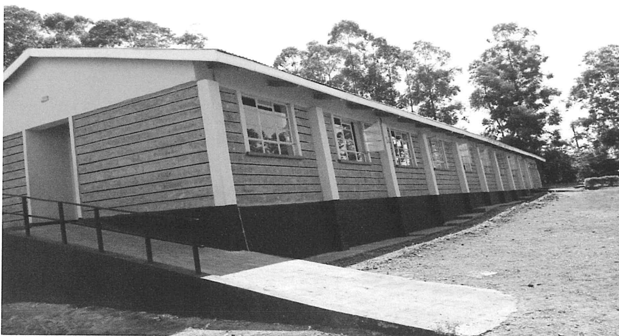
Fig 3: Shows a newly constructed 80 bed capacity dormitory at Lutacho Mixed Day and Boarding Primary School financial year 2019 – 2020 Webuye East Constituency for enhancing learning environment.
