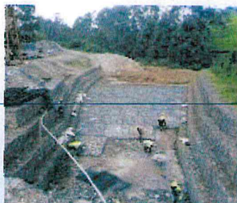
Githika Outfall Gabion Laying - (NCT)
