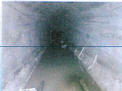
Lined Tunnel - Northern Collector Tunnel (NCT) Project
