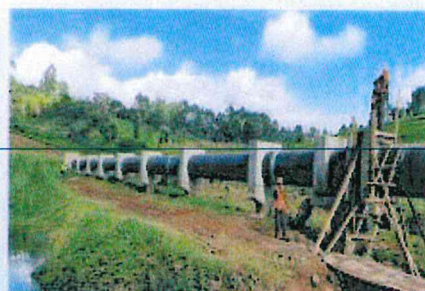
Aerial Crossing for NCT Pipelines project
