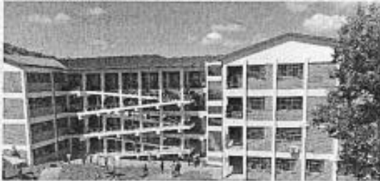
Newly Completed ADB Building
