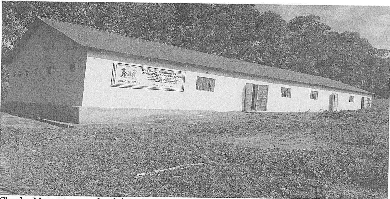
Chacha Moronge sec school dormitory
