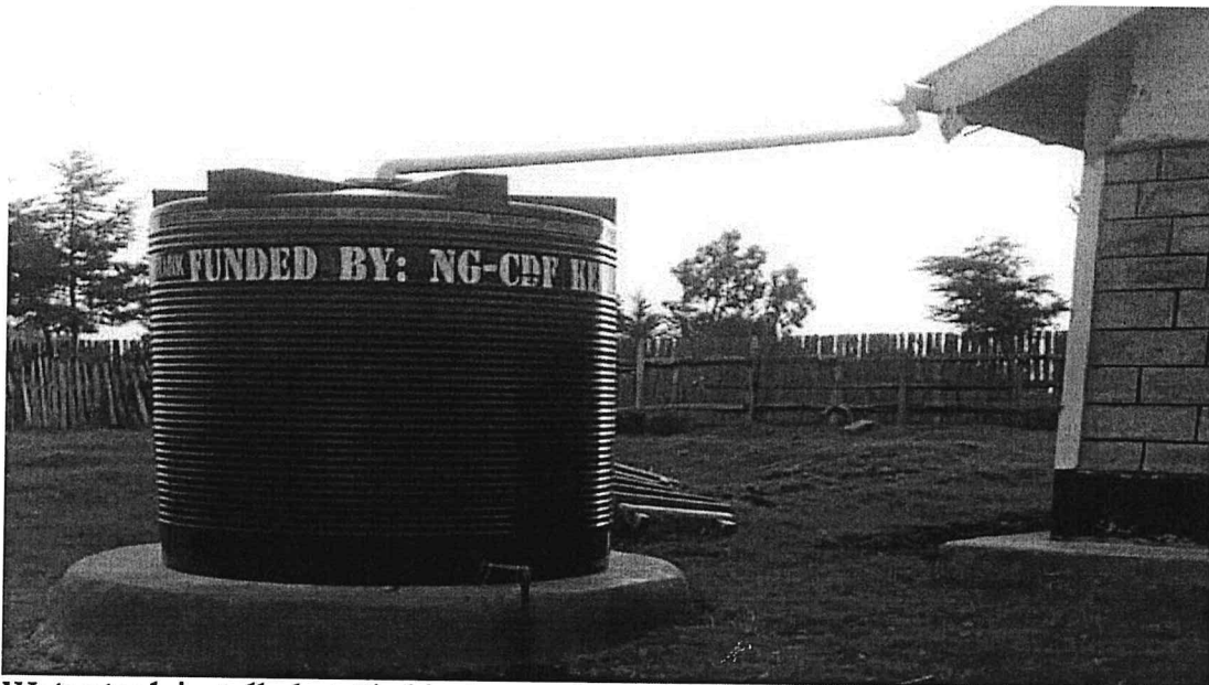
Water tank installed at Chebirei secondary school
