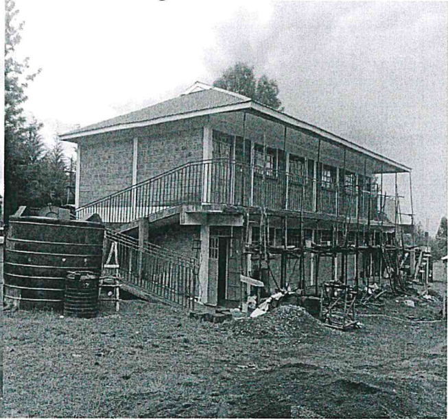
Ongoing 4No Classroom at St Patricks Secondary School
