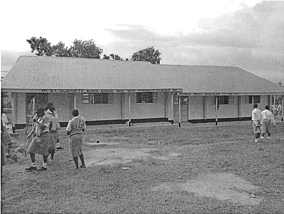
Diagram 1: St. Elizabeth Bumia Girls Secondary School – Construction of (2) two classrooms
