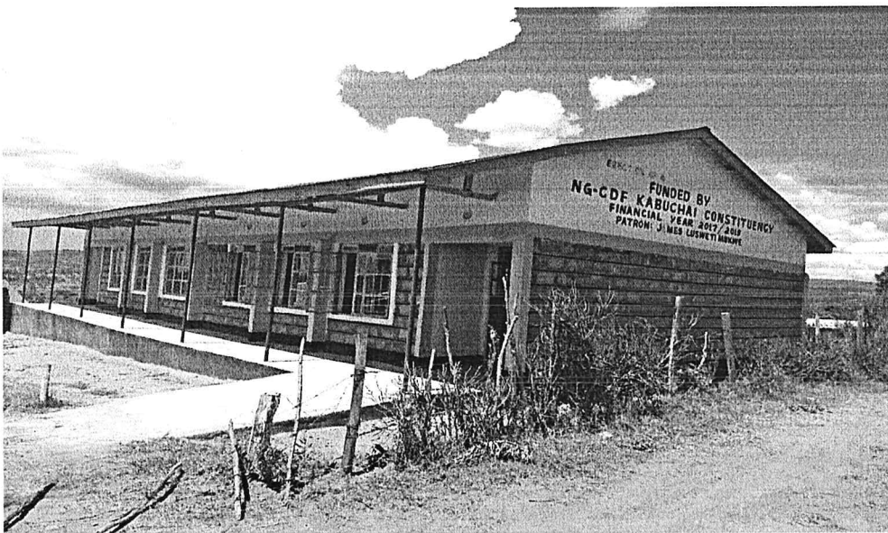
Chebunyi secondary school classrooms
