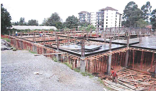
Construction of a four (4) level education tuition block complex.
