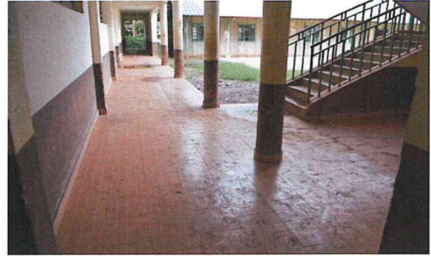
Block K Classroom Floor tiling
