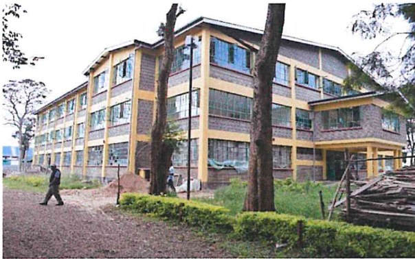
Phase II Construction of Electoral Engineering workshop
