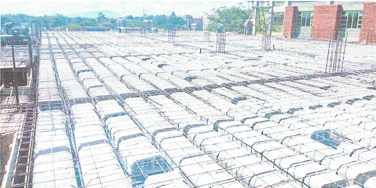
Slab construction - COETEC
