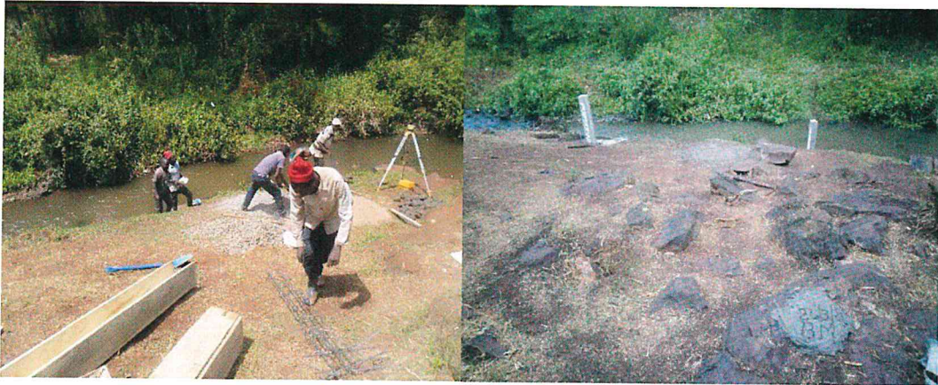
Figure 8: Rehabilitation at Kaptega River at Suam RGS 2B02A in Kapenguria
