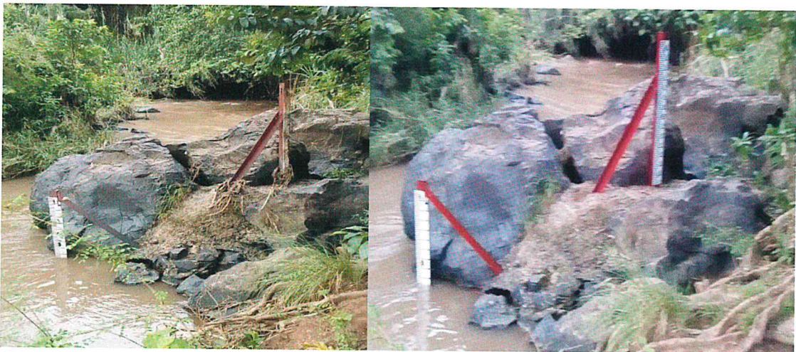
Figure 9: Rehabilitation at Awach Kajulu 1HA14 in Kisumu
