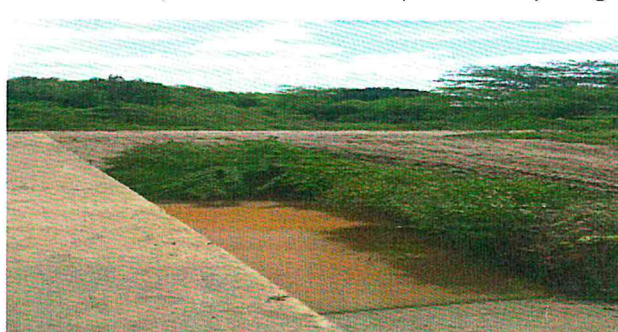
Repairs of the flood protection dyke section in at Mitapani breach at the preliminary stages
