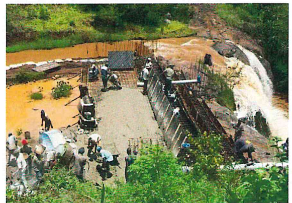
Gaitega Gatari project-River diversion works during intake structure construction
