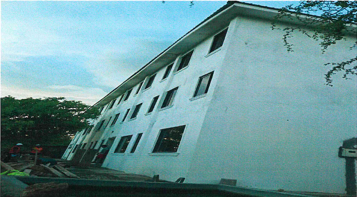
Newly constructed conference facility at Kilifi
