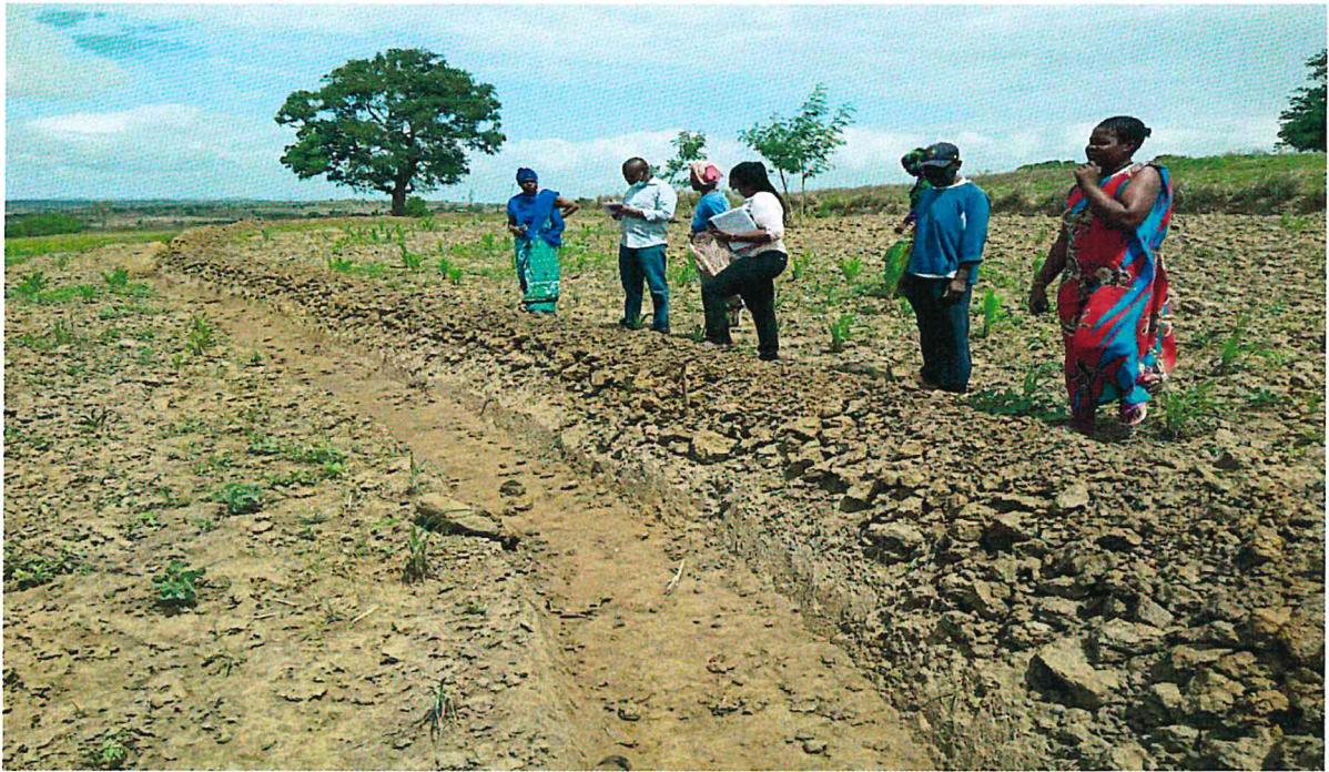
Ongoing terracing work at Mwache
