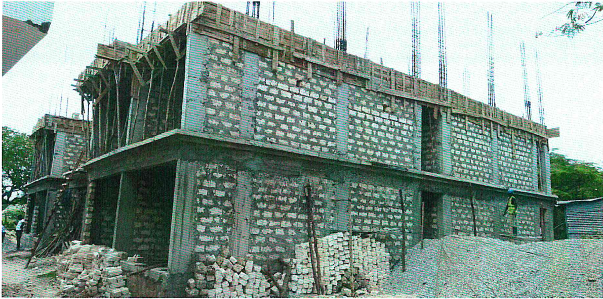
Construction of accommodation room in progress
