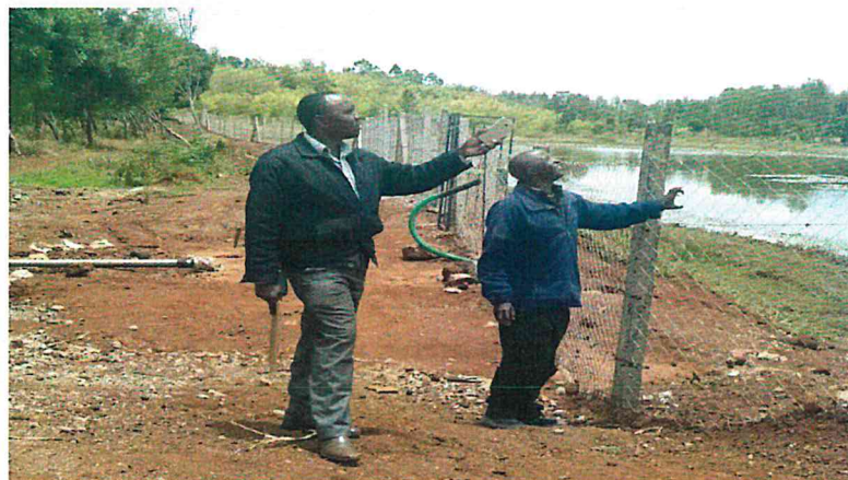
Overview of the Sama Mariki project showing the reservoir, fence and irrigation pipeline
