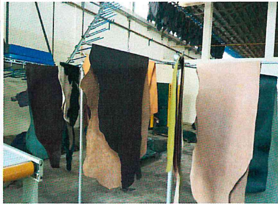
Installed overhead dryer
