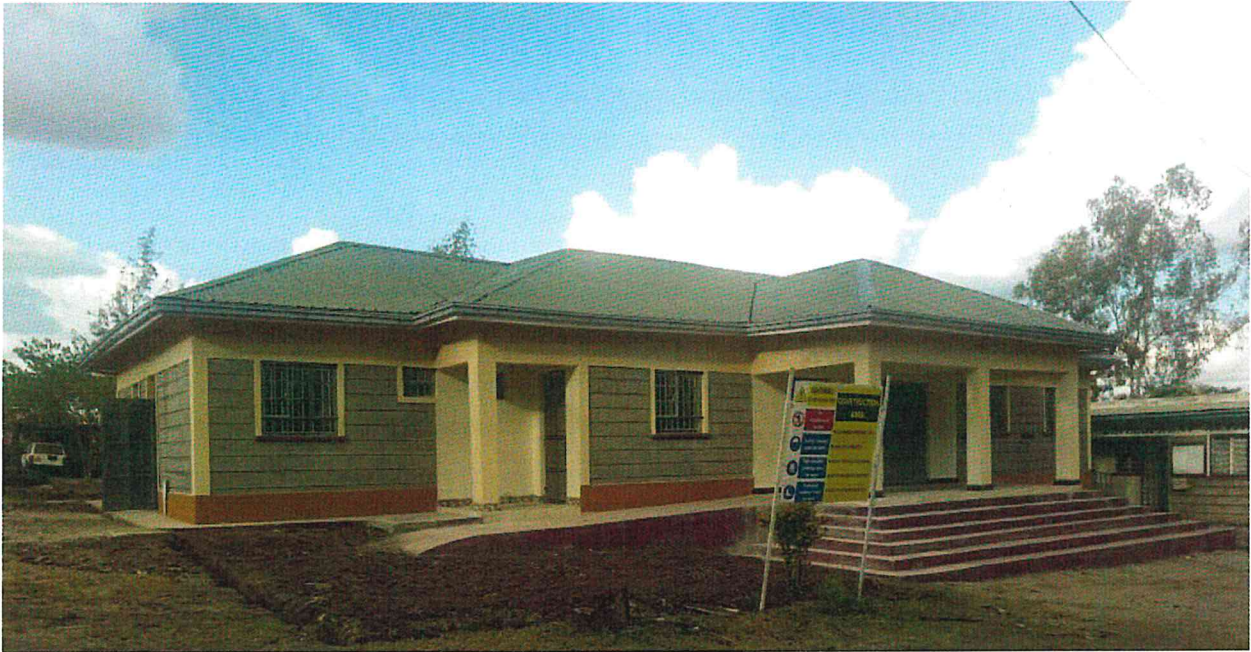
Newly constructed Samburu Office
