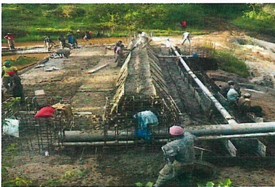
Gaitega Gatari Small Holder project water intake structure and pipeline installation works
