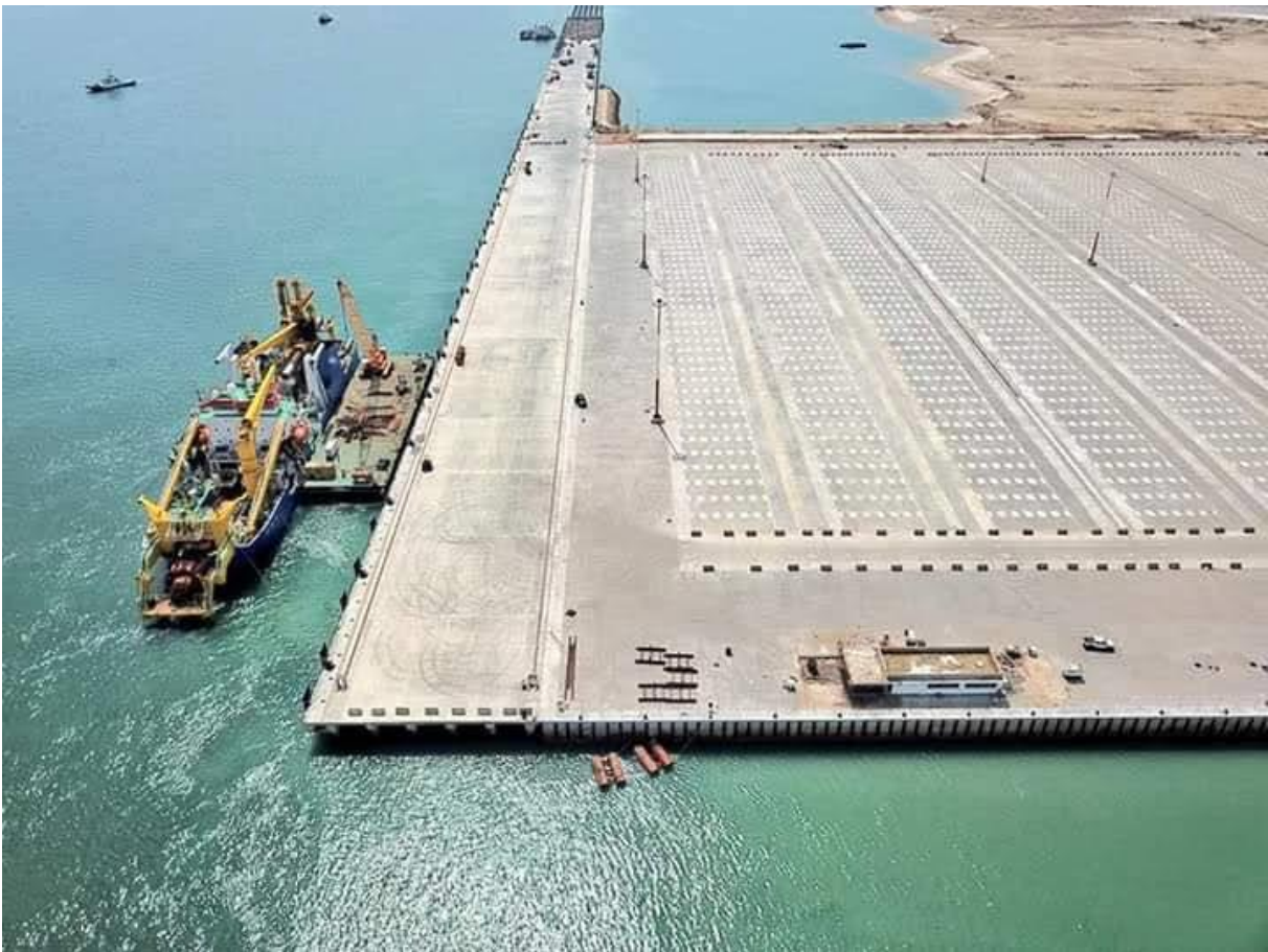
First Berth complete
